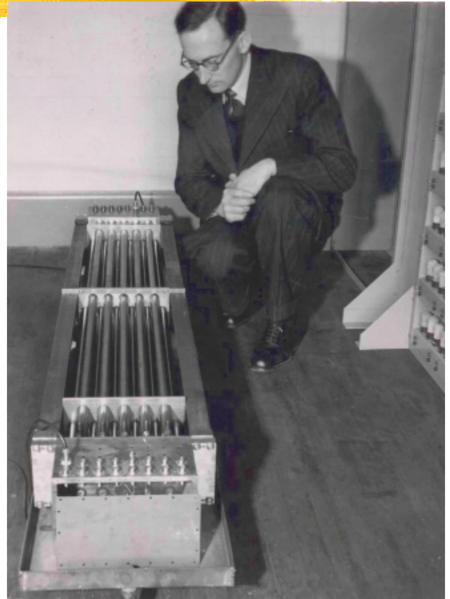
Memory Store: Mercury Delay Tanks
